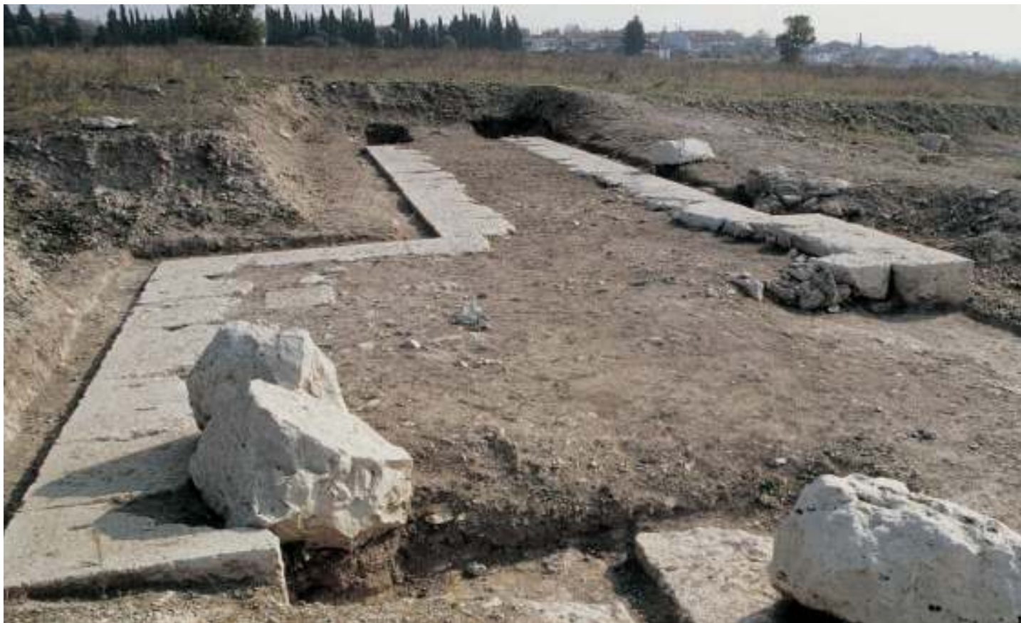
The defensive wall with a tower on the northwest part of the Palace hill.
