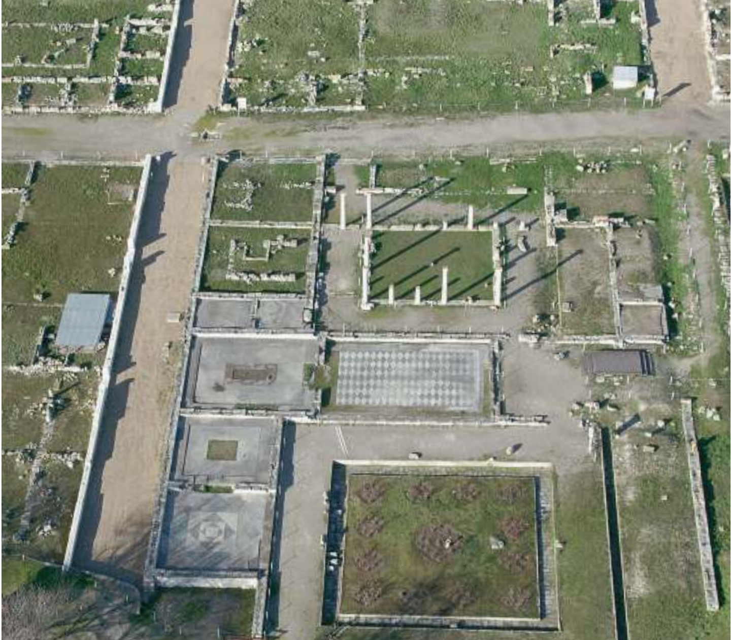
Aerial photograph of the house of Dionysos with the restored peristyle in the north courtyard.
