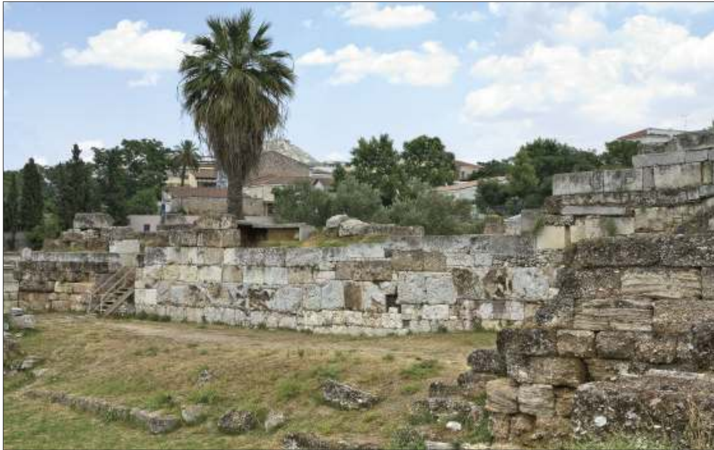
View from the Southwest of the Sacred Gate where successive phases of repairs to the fortifications may be clearly discerned.
