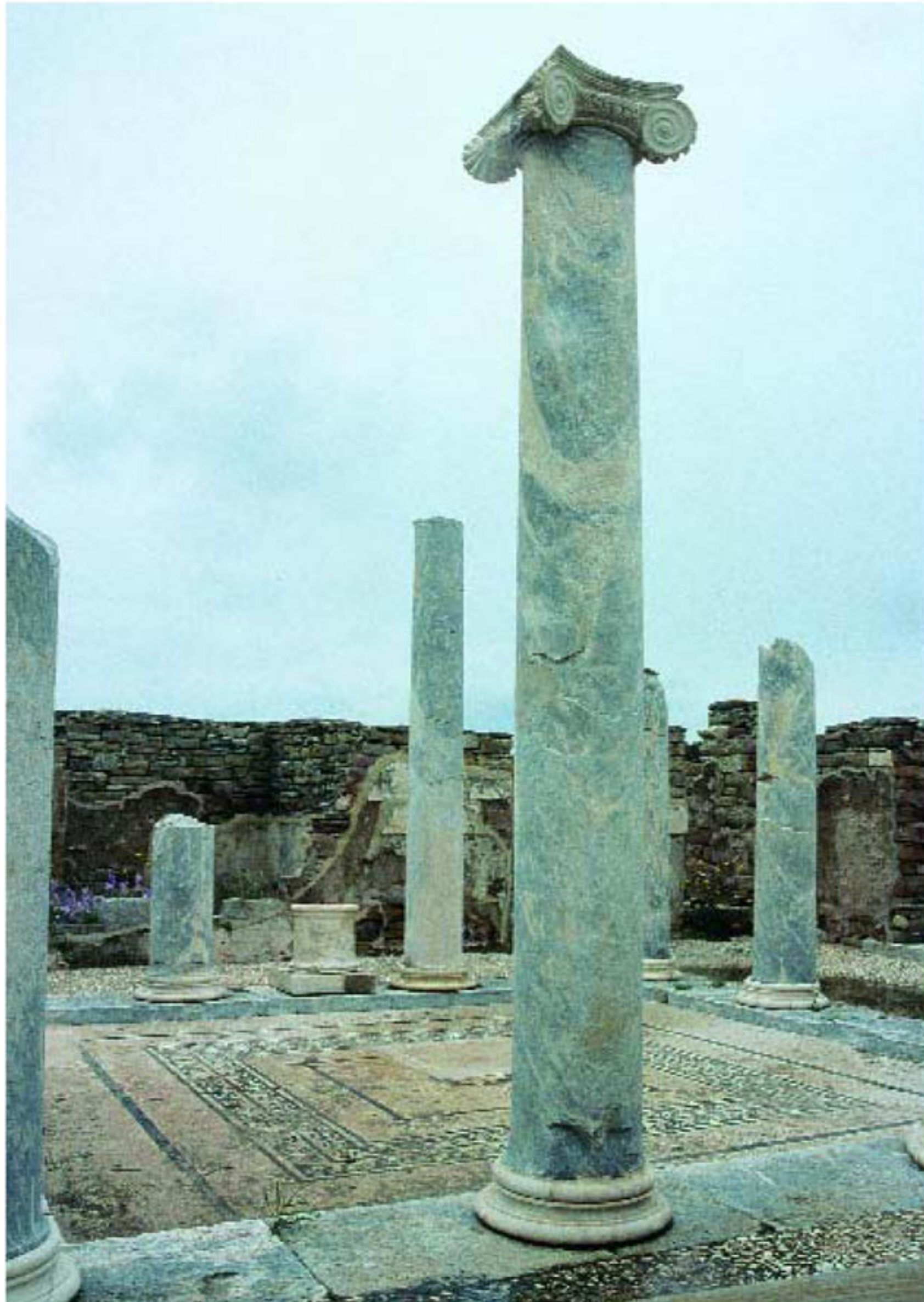
The peristyle of the Lake House has monolithic columns of grey-blue marble from Tinos, with bases and an especially decorative type of white marble Ionic capitals.
