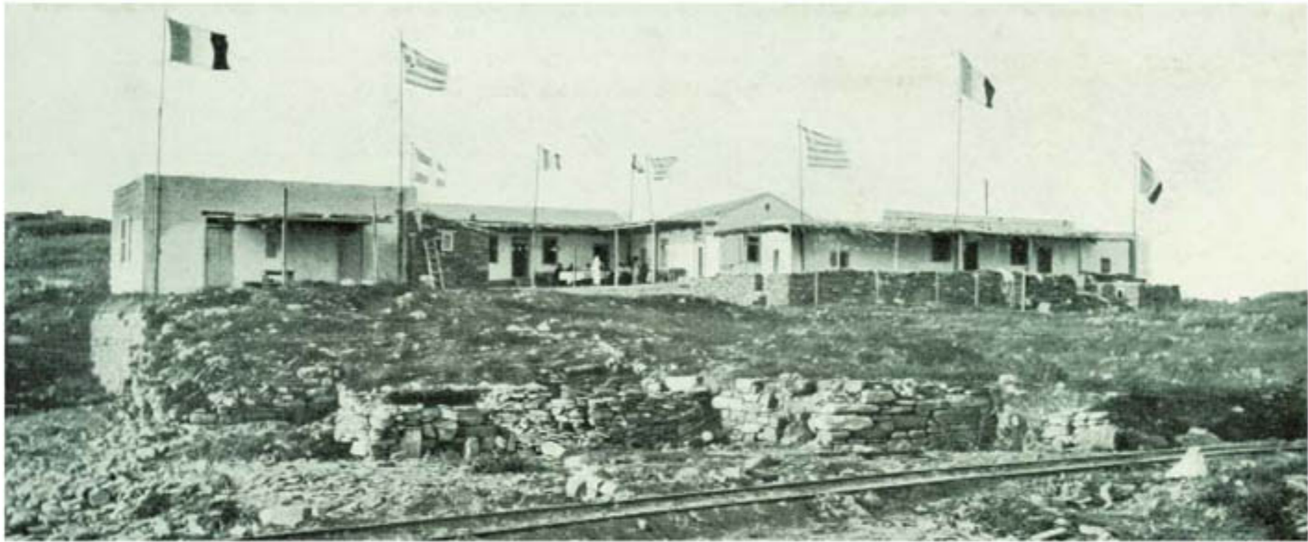
The French School celebrates Bastille Day on Delos. The School's building above the Hypostyle Hall is bedecked with flags on 14 July 1906. Below can be seen the rails for the wagons that dump the earth into the Sacred Port.
