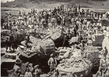
Large group of workers during the excavation of the Temple of Zeus (1875/76); Romaidis Brothers photograph.
